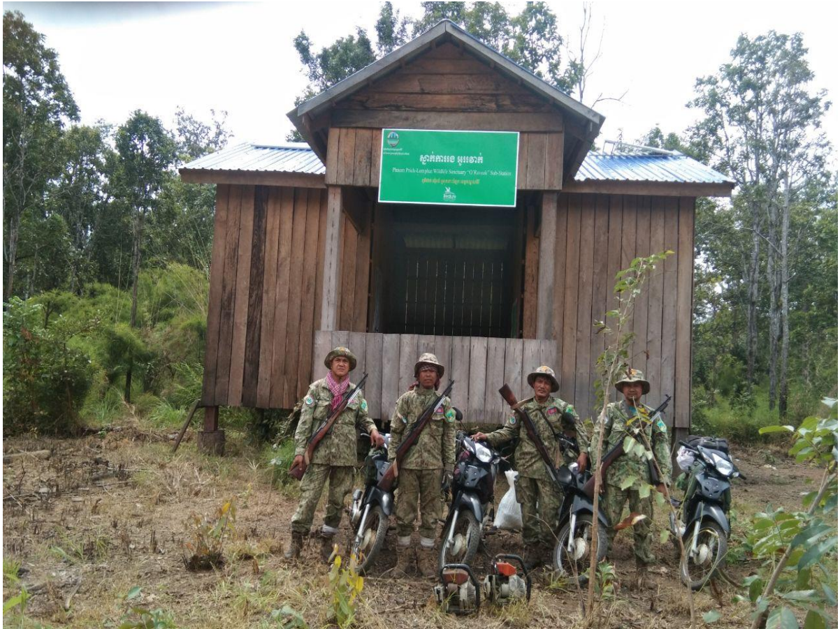
O'Roveak sub-station were built with financial support from BirdLife
