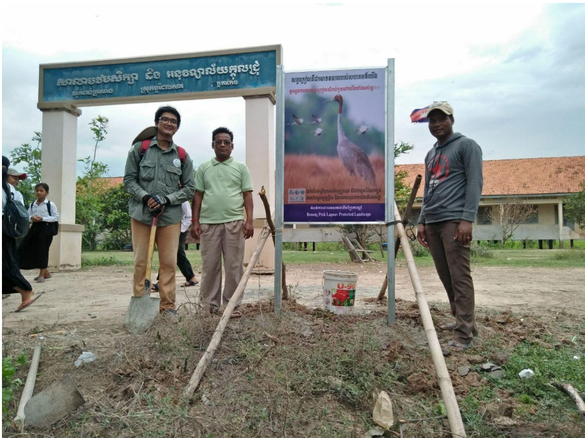
Installing signboard at school in BPL
