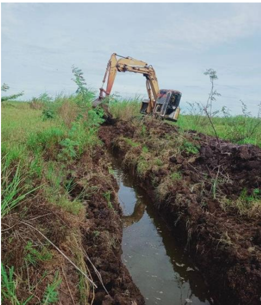
Figure 42. Blocking unused man-made ditches in BPL
